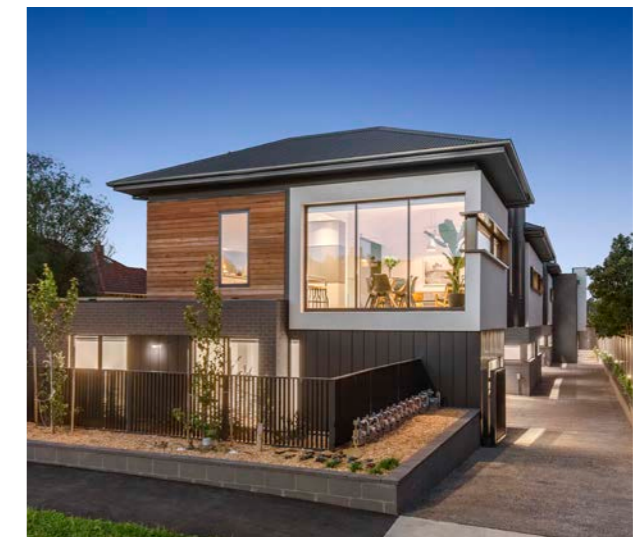
Photo of completed project
