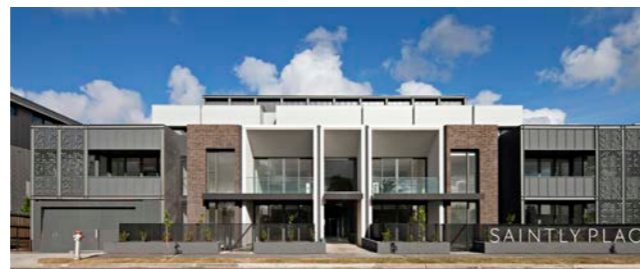
Photo of completed project
